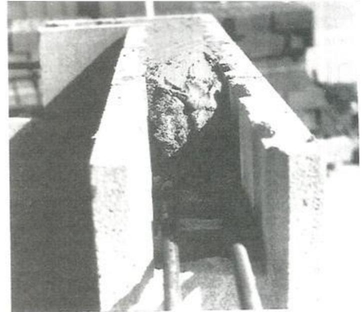
**Fig. 6-54.** Horizontal reinforcing bars positioned in a bond beam that will be solidly grouted.
