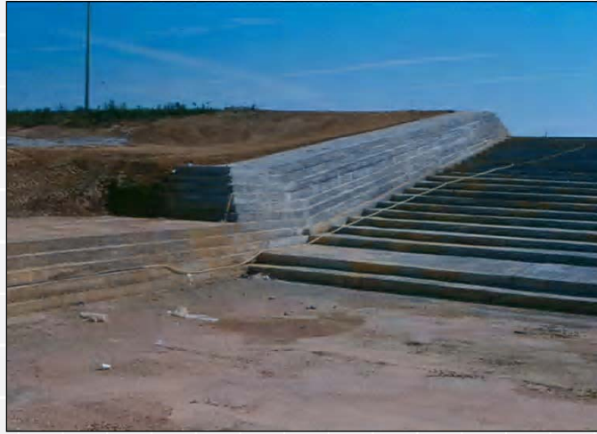
Lake Tholocco Dam – Alabama
