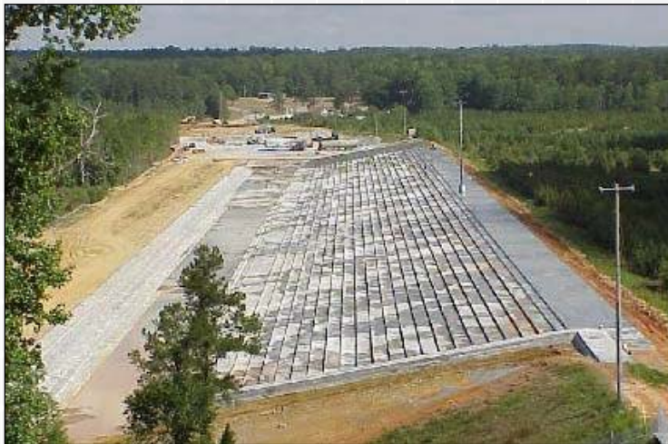
Lake Tholocco Dam – Alabama
