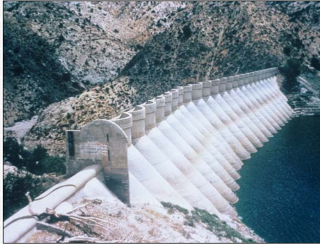
Littlerock Dam – California
