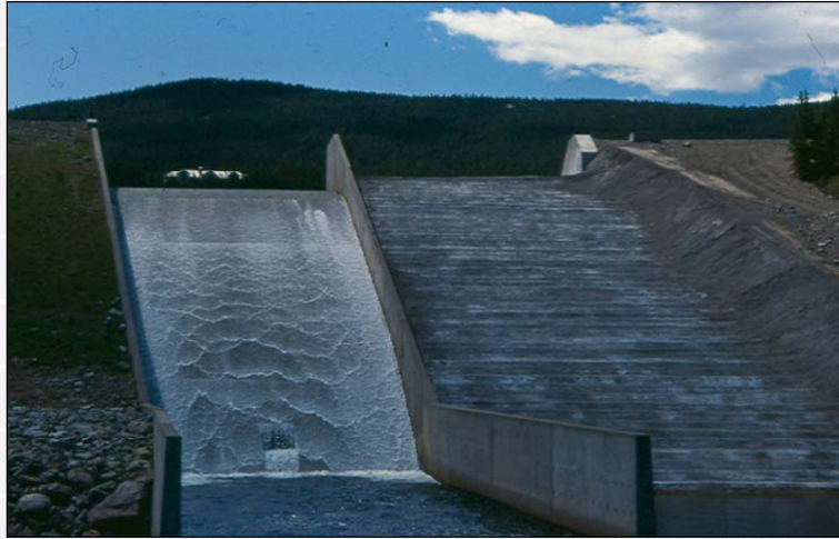
Goose Pasture Tarn Dam – Colorado
