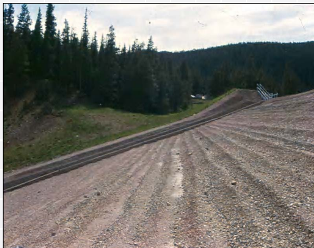
Spring Creek Dam – Colorado
