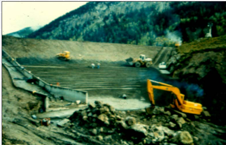
Spring Creek Dam – Colorado
