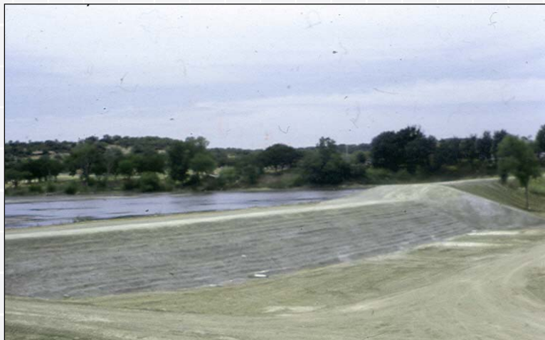
Brownwood County Club Dam – Texas
