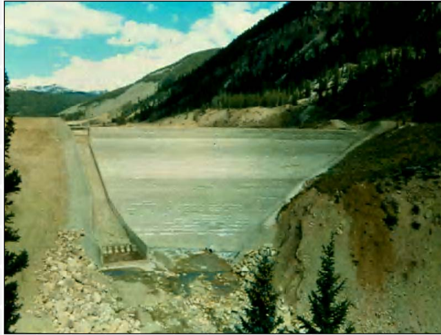
Spring Creek Dam – Colorado
