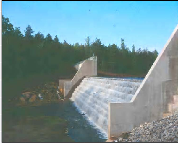
Towaliga Dam – Georgia
