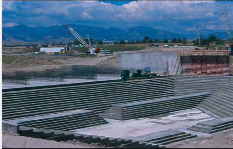
Standley Lake Dam – Colorado
