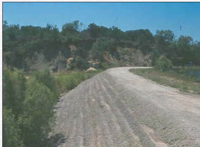
Brownwood County Club Dam – Texas
