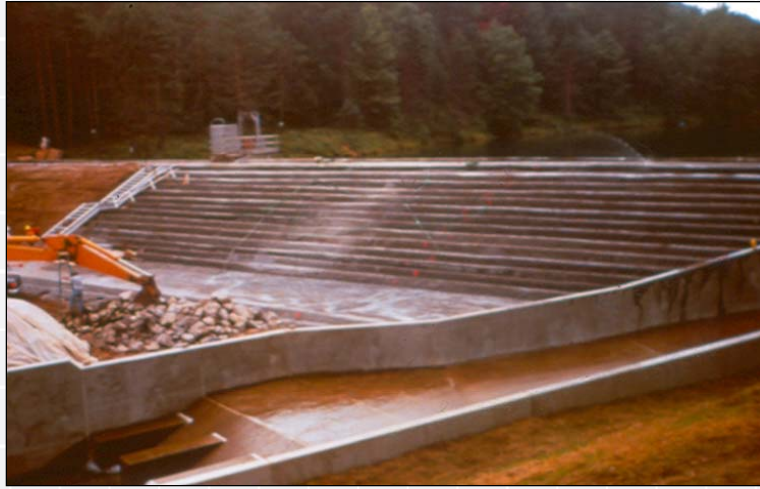
Phillipsburg No. 3 Dam – Pennsylvania
