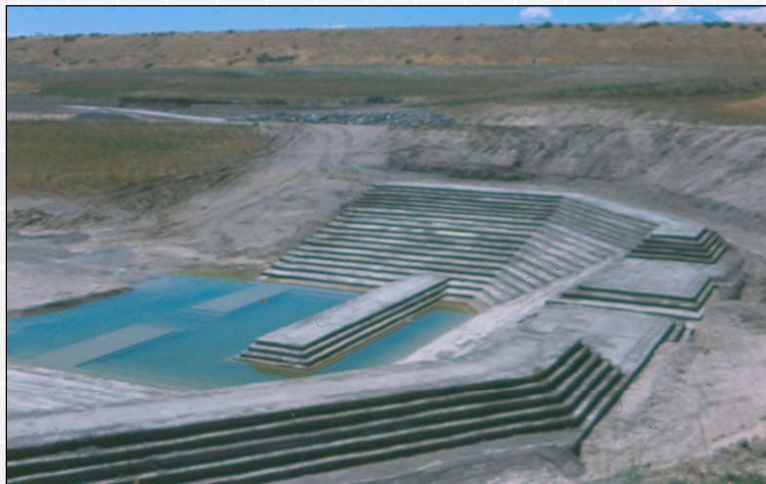
Standley Lake Dam – Colorado
