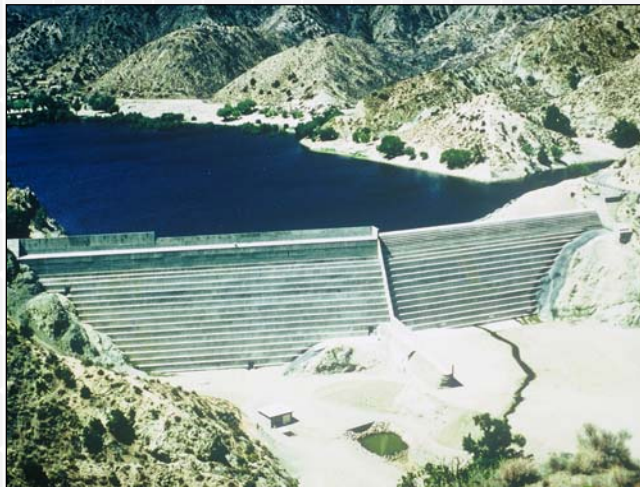
Littlerock Dam – California
