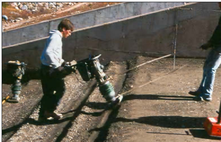
Goose Pasture Tarn Dam - Colorado
