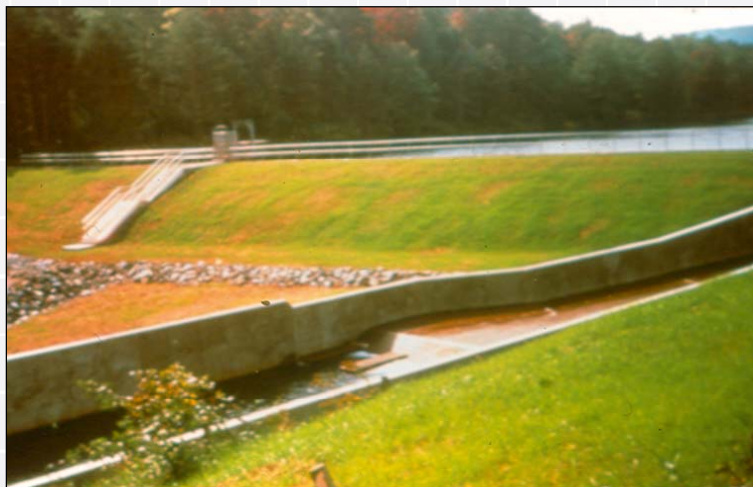
Phillipsburg No. 3 Dam – Pennsylvania
