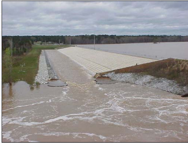
Lake Tholocco Dam – Alabama
