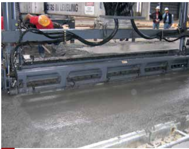
Extendidora laser screed .
